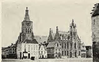
Dixmuiden. The Town Hall, 1914
